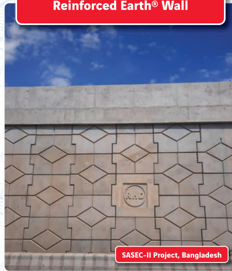
Reinforced Earth® Wall
